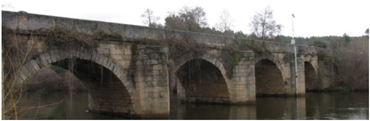
Bridge over the Tua (Mirandela)
