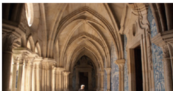
2. Cathedral of Porto (Porto) 3. Cloister of the cathedral of Porto (Porto)
